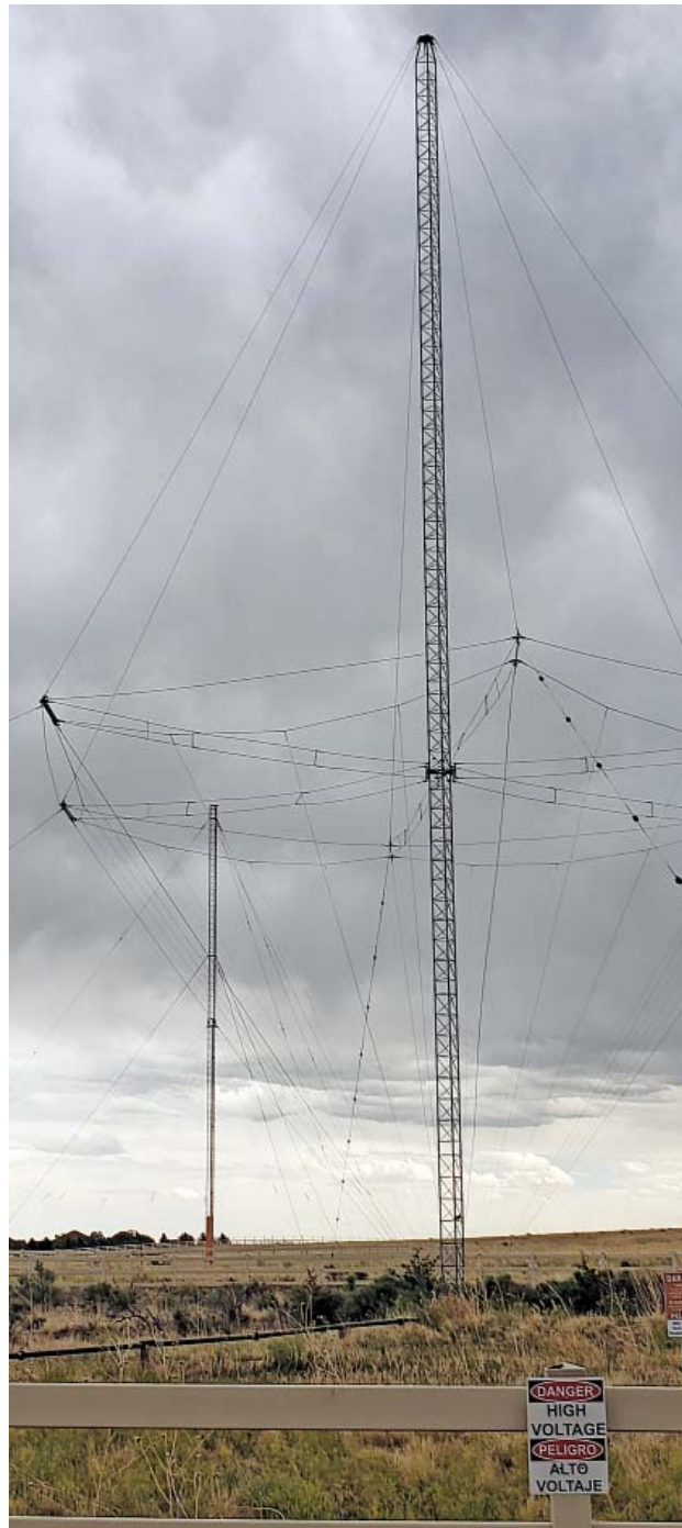
Figure 1 — The antenna in the foreground is a standby broadband antenna with an inverted cone design. It can operate at any of the WWV frequencies from 2.5 to 25 MHz. The primary 5 MHz antenna is in the background.
