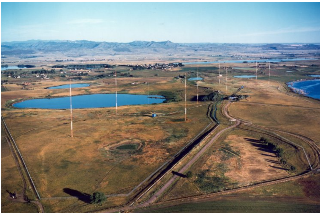
Fig. 24. Aerial view of WWVB, looking northwest.
