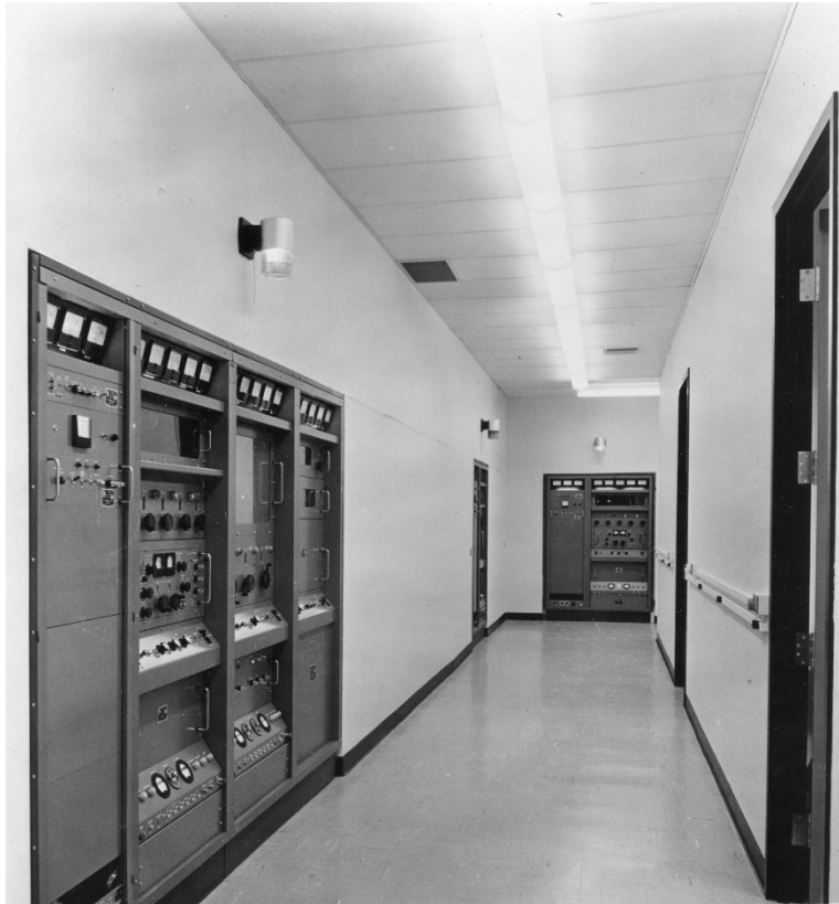
Fig. 19. Interior of WWV building in Fort Collins, Colorado, 1966.
