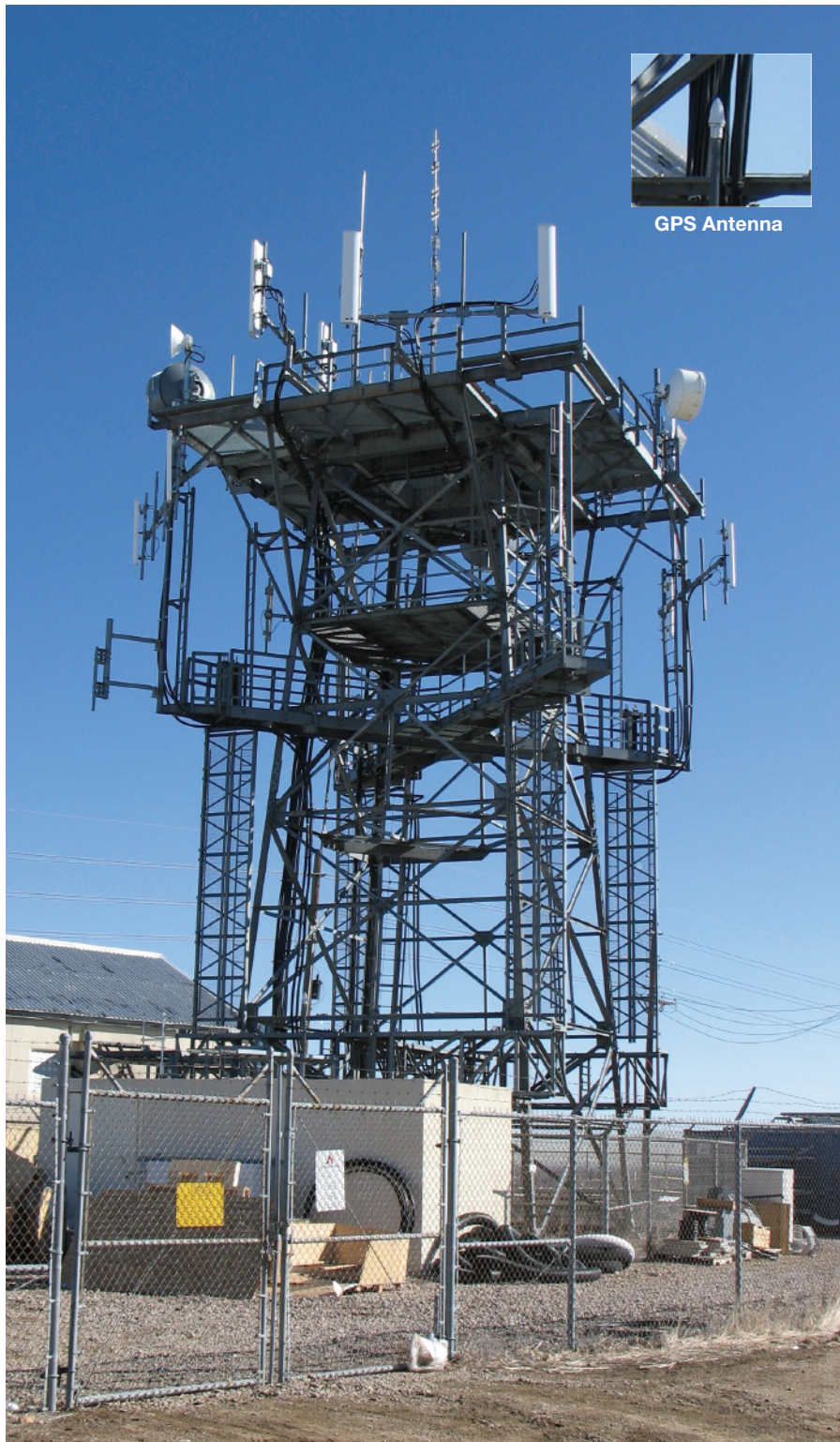
Figure 5. Cellular telephone towers contain a myriad of antennas, often including GPS antennas used to obtain a CDMA time reference.
